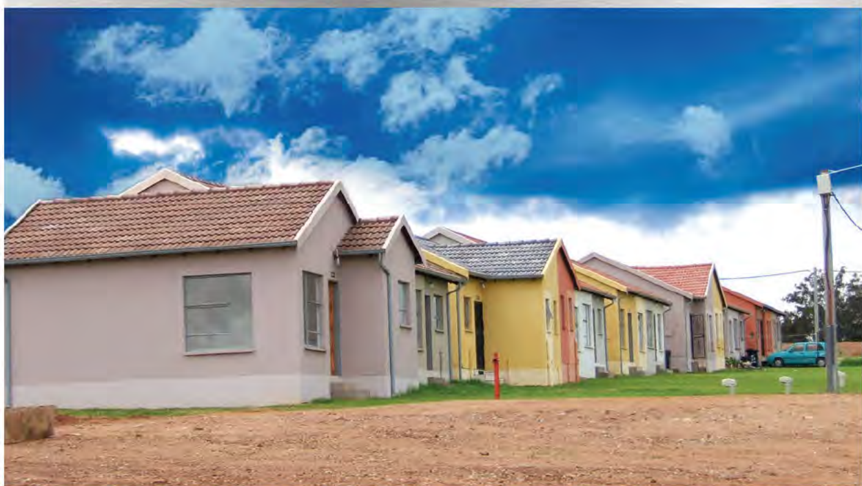
Affordable homes built with investments from the OPIC-supported South African Workforce Housing Fund are providing housing to nearly 8,000 low-income and working class families in Johannesburg.
