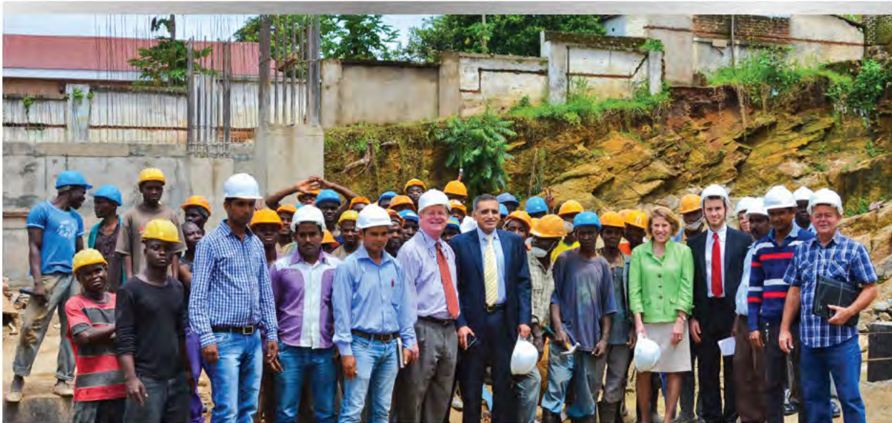
OPIC President and CEO Elizabeth Littlefield visits a construction site in Malawi, one of several countries she visited in 2014 to explore investment opportunities.
